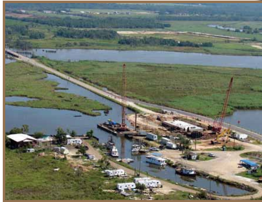
Aerial view of the project area.
