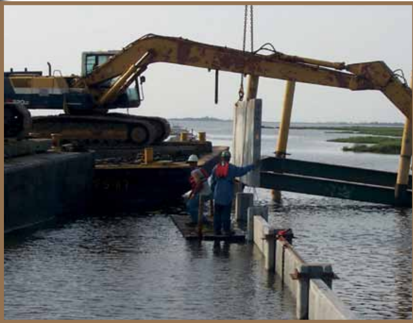
Panel structures being used for a field test.
