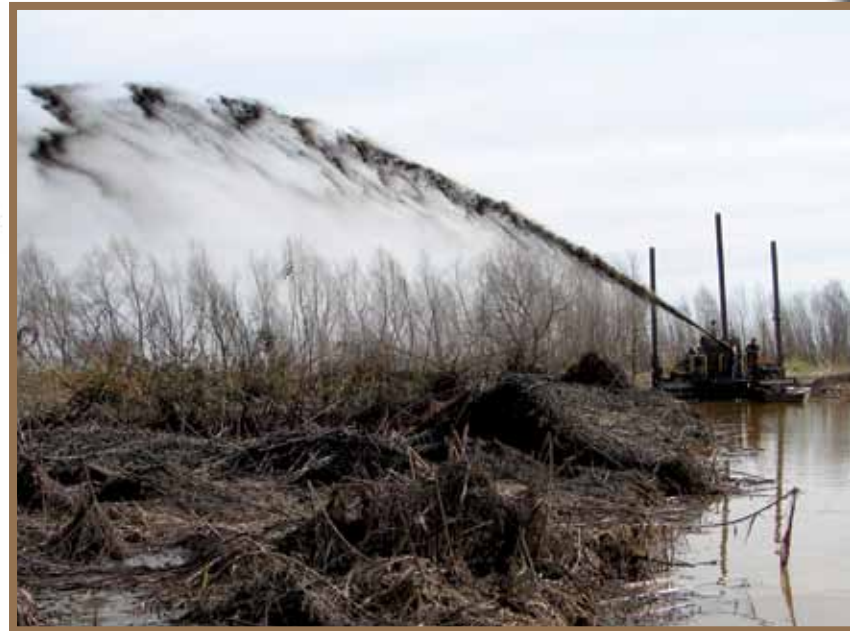
Spray dredging is used to rebuild marshes.
