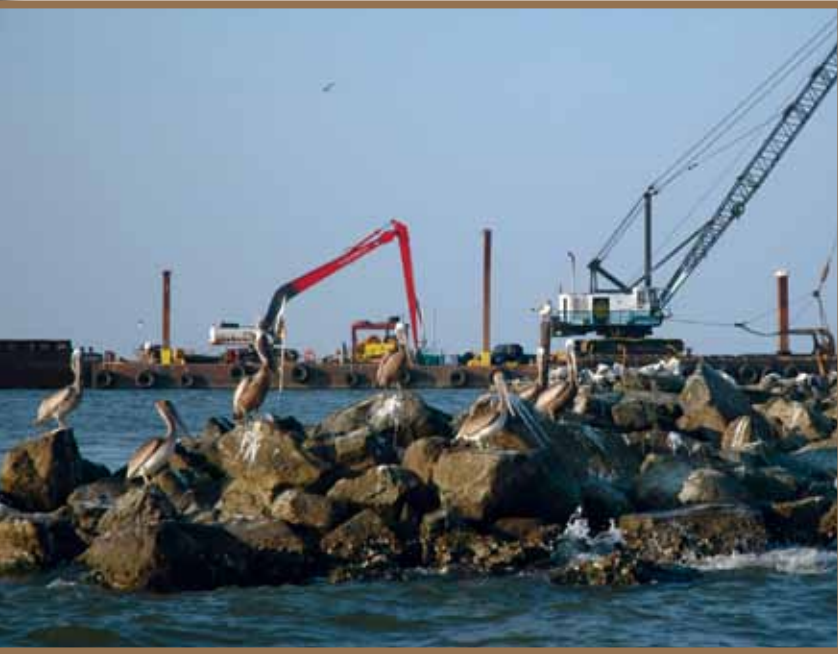
Construction crews build breakwaters on Raccoon Island.
