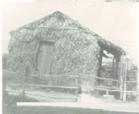
Palmetto houses were common throughout coastal Louisiana in the 19th century. (National Archives)
