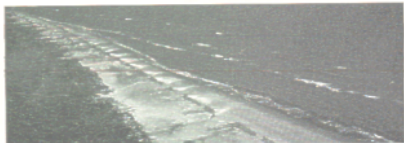
Sediment-trapping fences line the shore at Timbalier Island. (DNR Photo)
