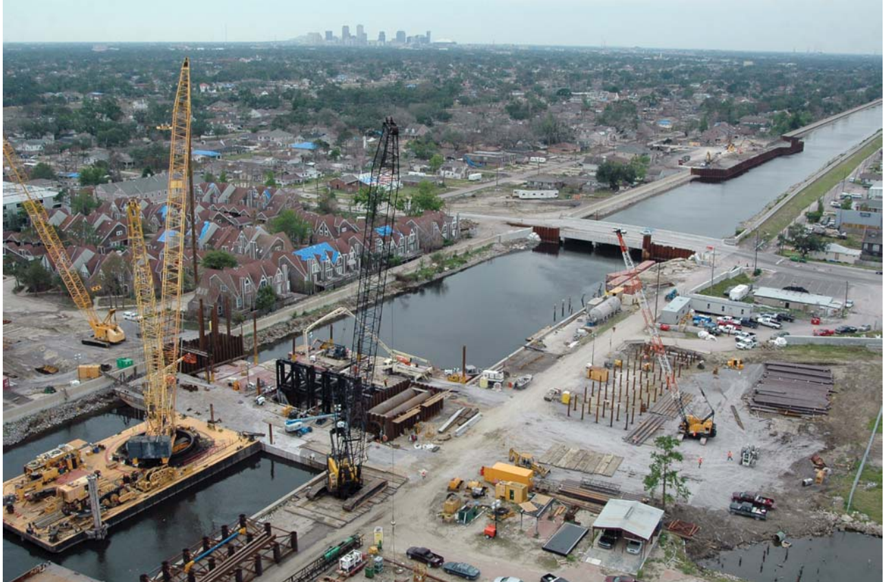
In the year following Katrina's landfall, efforts to restore Louisiana's hurricane protection system included building improved floodwalls and installing temporary floodgates and additional drainage pumps. State and federal agencies are working to strengthen southern Louisiana's capability to endure severe storm conditions by combining flood protection with coastal restoration.
