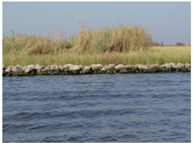
A mature, self-sustaining marsh flourishes behind a rock barrier. Such barriers will encourage the stabilization of Lake Boudreaux project areas by protecting them from wave-induced erosion.
