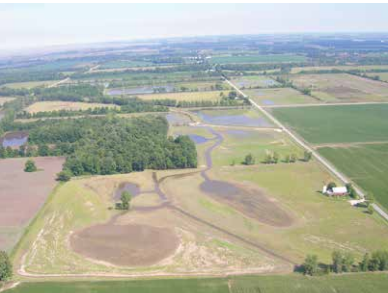
Project area immediately after construction.
